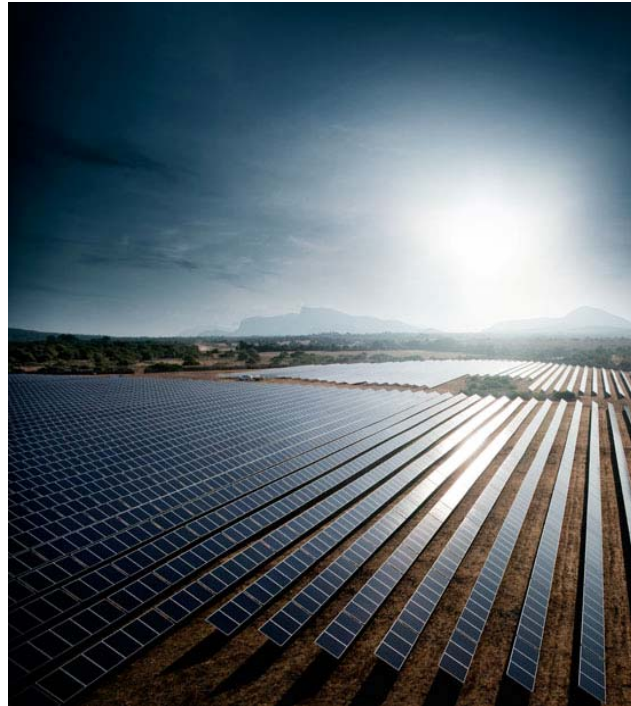
Figure 3-4. Typical 1 MW Capacity Fixed Tilt Solar System
